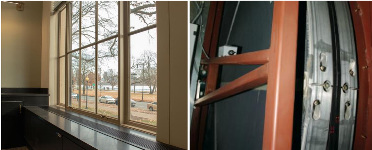
Figure 5: Left: Vacuum insulation glass was used to replace the single pane glazing units in Building 2 (Photo credit: E. Reinhard); Right: Energy Recovery Ventilation (ERV) enthalpy wheel in Building E62 (Photo credit : M. Craven, MIT)
